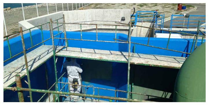
This desalination plant in Cyprus required long term substrate protection against raw salty sea water in the primary collection tanks and a lining that was suitable for storing potable drinking water once the water had been desalinated and refined.
