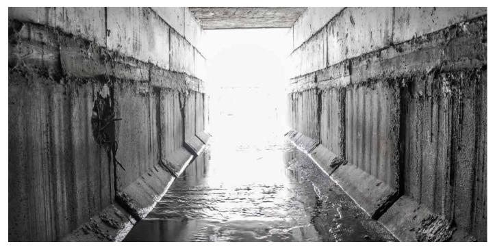
The Water and Sewerage Authority of the Punjab province in Pakistan required a high performance lining solution to protect new under road sewage tunnels. The "cut and fill" construction method required an external coating that could provide impact protection against back filling operations and survive a life time buried under the road.
