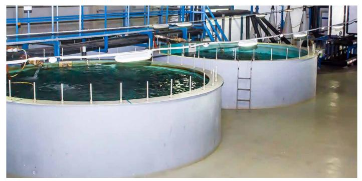
Marine Harvest a leading fish farming company required a tank lining system that would protect the internal tank surfaces, be easy to clean and provide a smooth surface that would not damage the fish.
